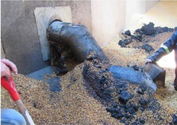
Aeration transitions inspected for damage and repaired
