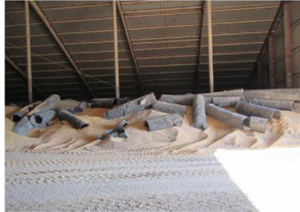
Air tubes inspected for damage and repaired
