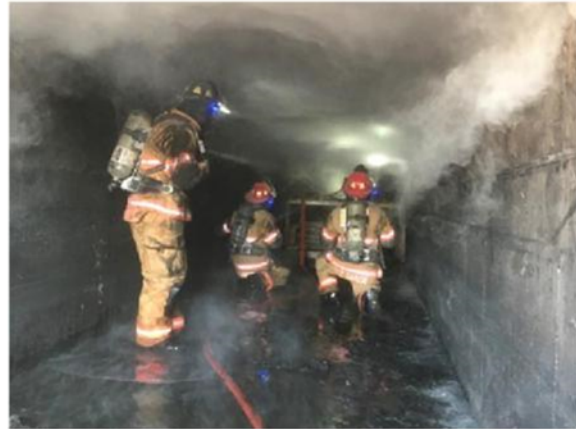
Out of condition grain caused reclaim conveyor belt in tunnel to burn
