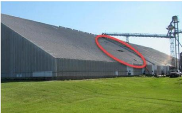
Holes cut for access to fire or smoke venting repaired
